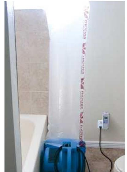
**Air mover with ducting connected to Exhaust Controller**
