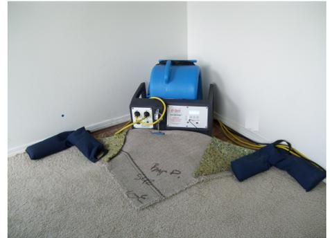
**Step #4 - Reduction of vapor saturation levels (humidity) by dehumidification or evacuation (Dehumidification)**
