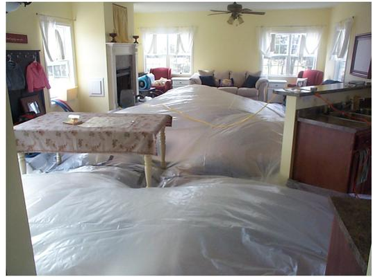
**Step #3 - Airflow applied directly to the water (Evaporation)**
